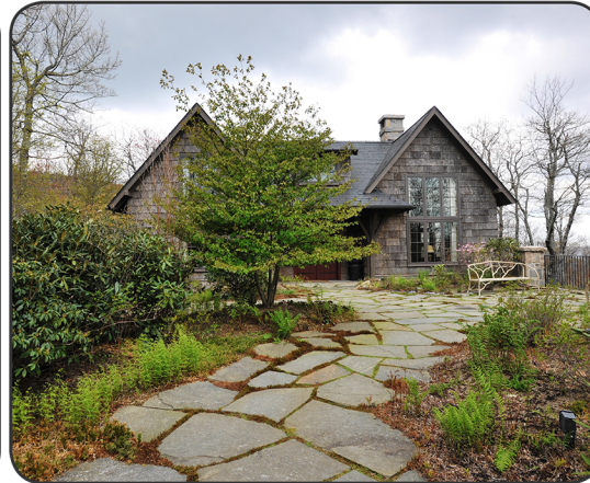
INTENSIVE GREEN ROOF
